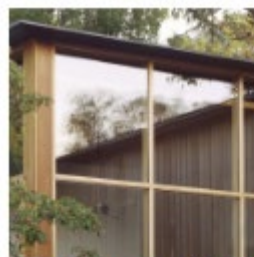
7 Aluminium Framed Glazing TIMBER COLOURED
