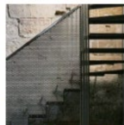
8 Metal Mesh Balustrade POWDER COATED: DULUX ELECTRO VENERABLE SILVER KINETIC
